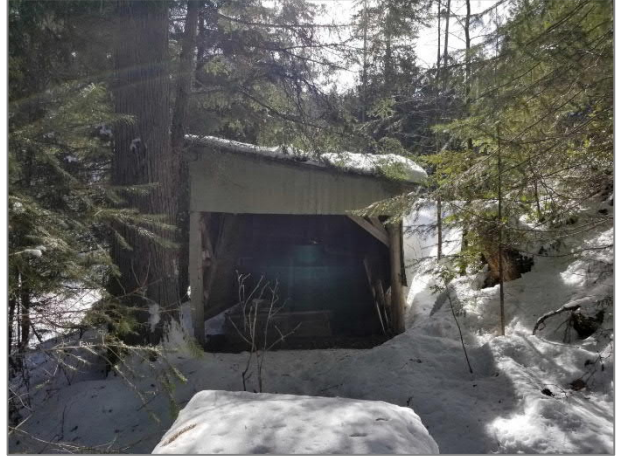
Photo 4. Domestic water system pumphouse structure, located just upstream of the proposed bridge crossing.
