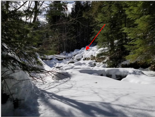
Photo 5. View of armoured rock bank upstream of bridge crossing and pump house.
